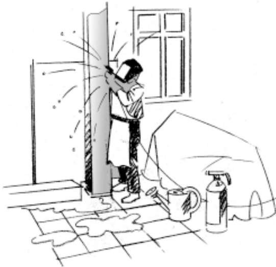
Fig. 10. It is important to protect fire sensitive things where there is risk of fire when welding.
